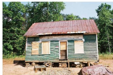
This photo shows the slave cabin resting on the original rock piers in its new home at the Nacoochee Valley African American Heritage Site & Nature Preserve. Stone mason David Vandiver will reassemble the rock chimney and hearth. Photo by Jeanne Cyriaque
