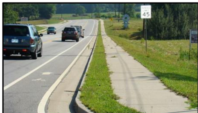
Figure 7. Bike Lanes and Sidewalks along GA Hwy 75
